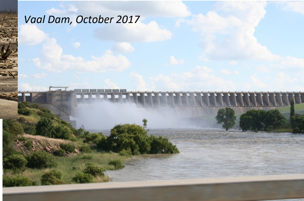
Image credit: Infrastructure News
