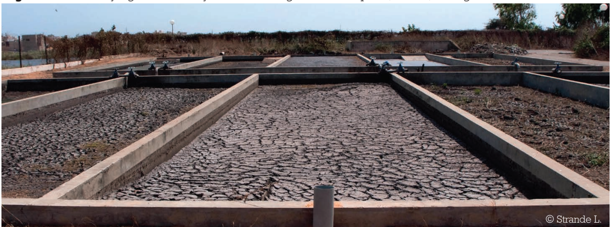
Figure 2.3.3. Drying beds at Niayes faecal sludge treatment plant, Dakar, Senegal.
