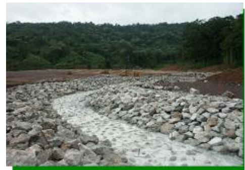
Figure 4: Drainage system in one of the working sites
