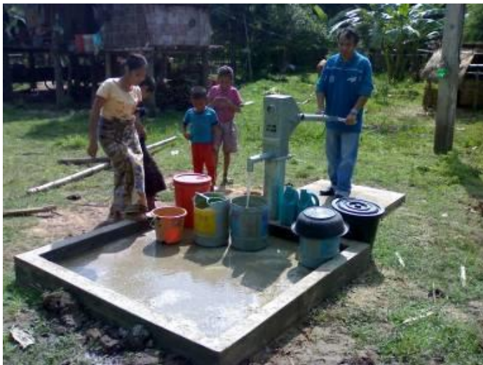
Figure 7: one of the 500 boreholes equipped with Afridev pump
