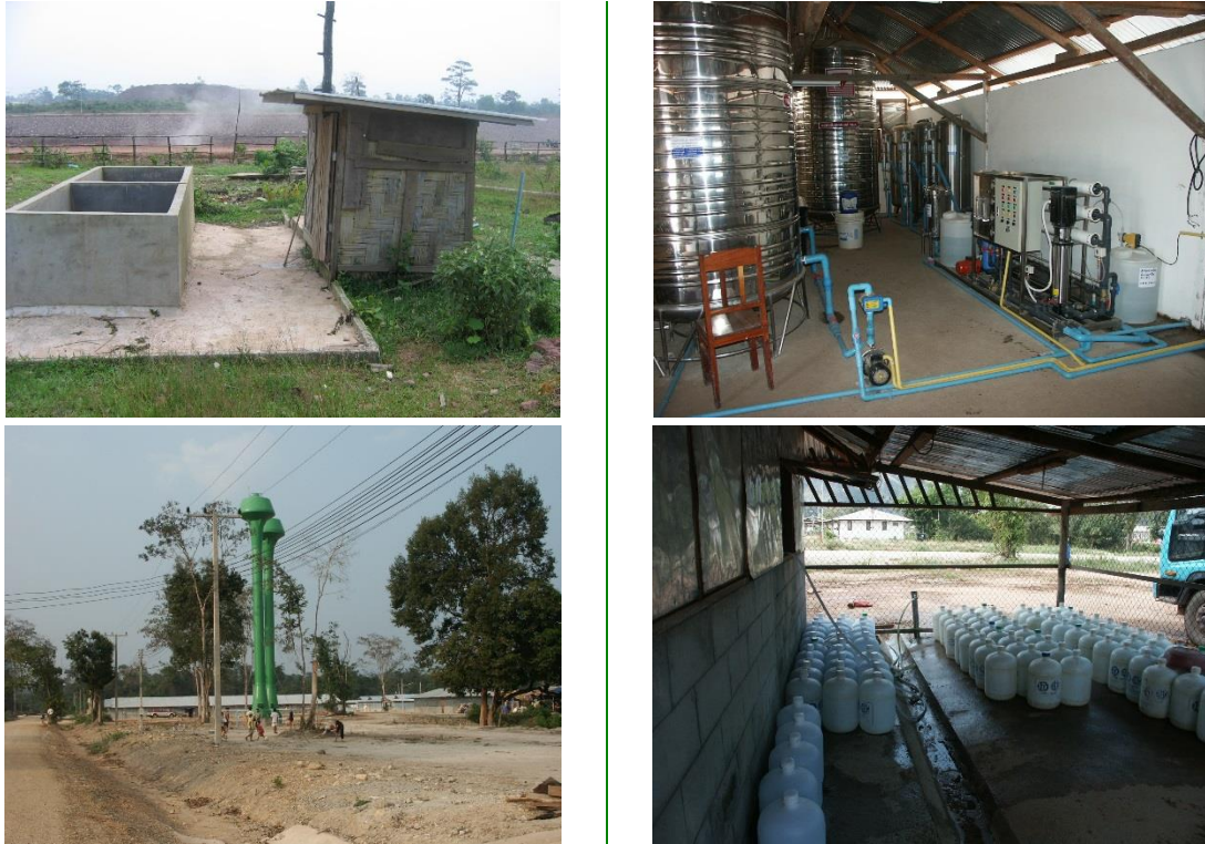
Figure 6: (a) Top left-hand picture: toilet (right) and water container for washing and personal hygiene purposes (left); (b) Top right-hand picture: drinking water treatment plant in the main camp; (c) Bottom left-hand picture: water tower in the main work camp – as a direct drinking water source for the main camp and an indirect one for secondary camps (to which drinking water is transported via trucks and water tanks, see picture d); (d) Bottom right-hand picture: water tanks for transporting drinking water from the main camp to secondary work camps.
