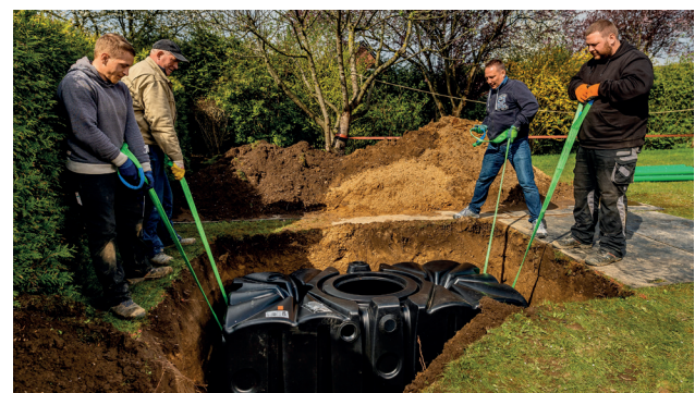
Installation of a Rainwater Harvesting Tank
