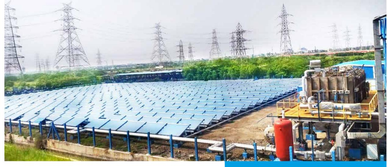
M<sup>2</sup> Area, 600 KWth at GHI 600 W/M<sup>2</sup>) is flashed in a chamber, which is maintained under vacuum to generate low-pressure steam. During non-solar/ low solar period, heat of auxiliary steam will be utilized for MED. LP steam heat exchanger is used for this purpose.
