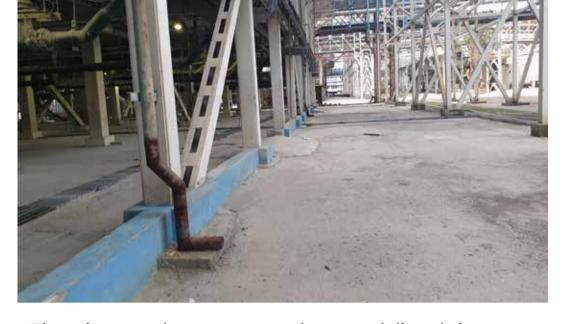
The rainwater down comers to be routed directly into storm water drain which finally goes out of the facility without any treatment.
