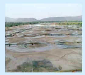
Reuse of water for Dust Suppression in Ash pond
