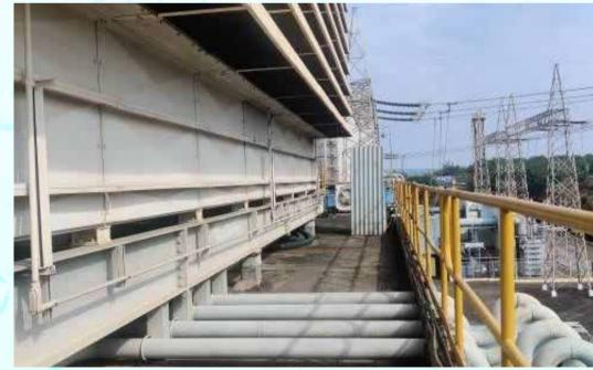
Inlet Air Chiller Coil condensate Collection lines
