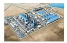
Al Dur: the largest desalination plant with Reverse Omosis technology in the Middle East Al Dur, in Bahrain, is the largest Seawater Reverse Osmosis plant drawing water from the Gulf with a capacity of 218,208m3/d and 1,234MW of power production. It is a potent symbol of the acceptance
