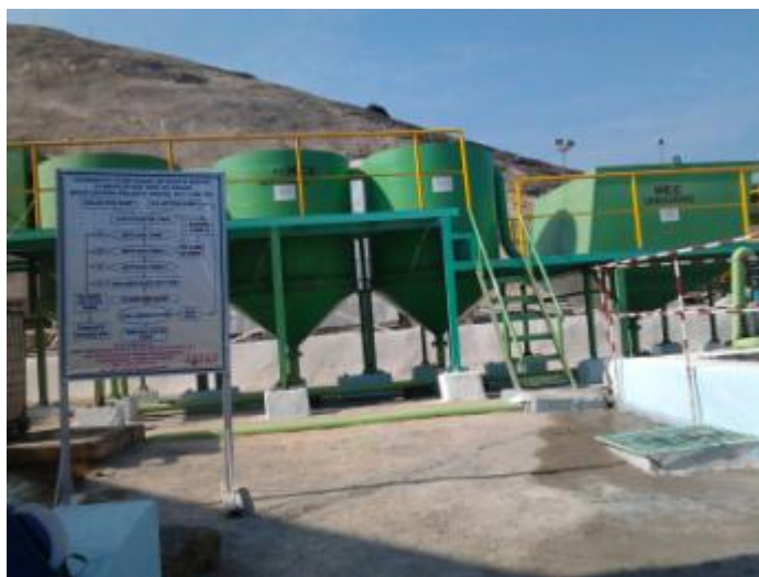
Wastewater treatment plant for tunnel wastewater
