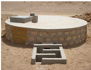
Tanka: Cylindrical well for drinking water
