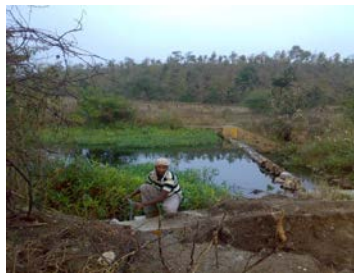
Phad: Small-scale community-led diversion for irrigation
