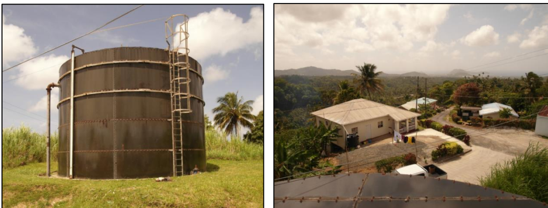
Treated water storage – Trigo
