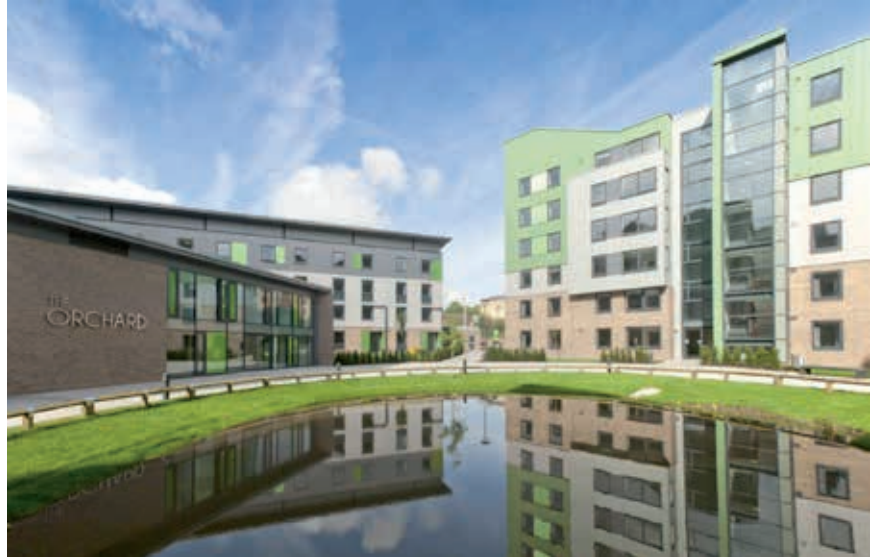
↑ The Green, an eco-friendly student accommodation at the University of Bradford in the UK, was built with solutions from British Gypsum and Saint-Gobain ISOVER.
