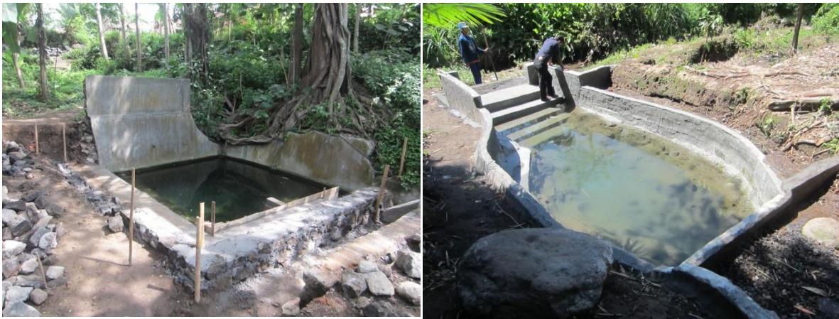
Two water sources in Soran Village, Umbul Gendruwo and Umbul Ndoya, under construction. Both water sources are used for community daily activities including washing and drinking. Education on water hygiene and renovation of the water sources aim to ensure their sustainability.
