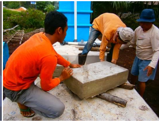
Water purification installment together with localcommunity
