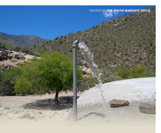
water and has freed more time for other tasks. Choosing to install an SQFlex pump means that the village is not dependent on electricity. The pump uses solar cells to operate which is essential in an area where electricity is a scarce resource.
