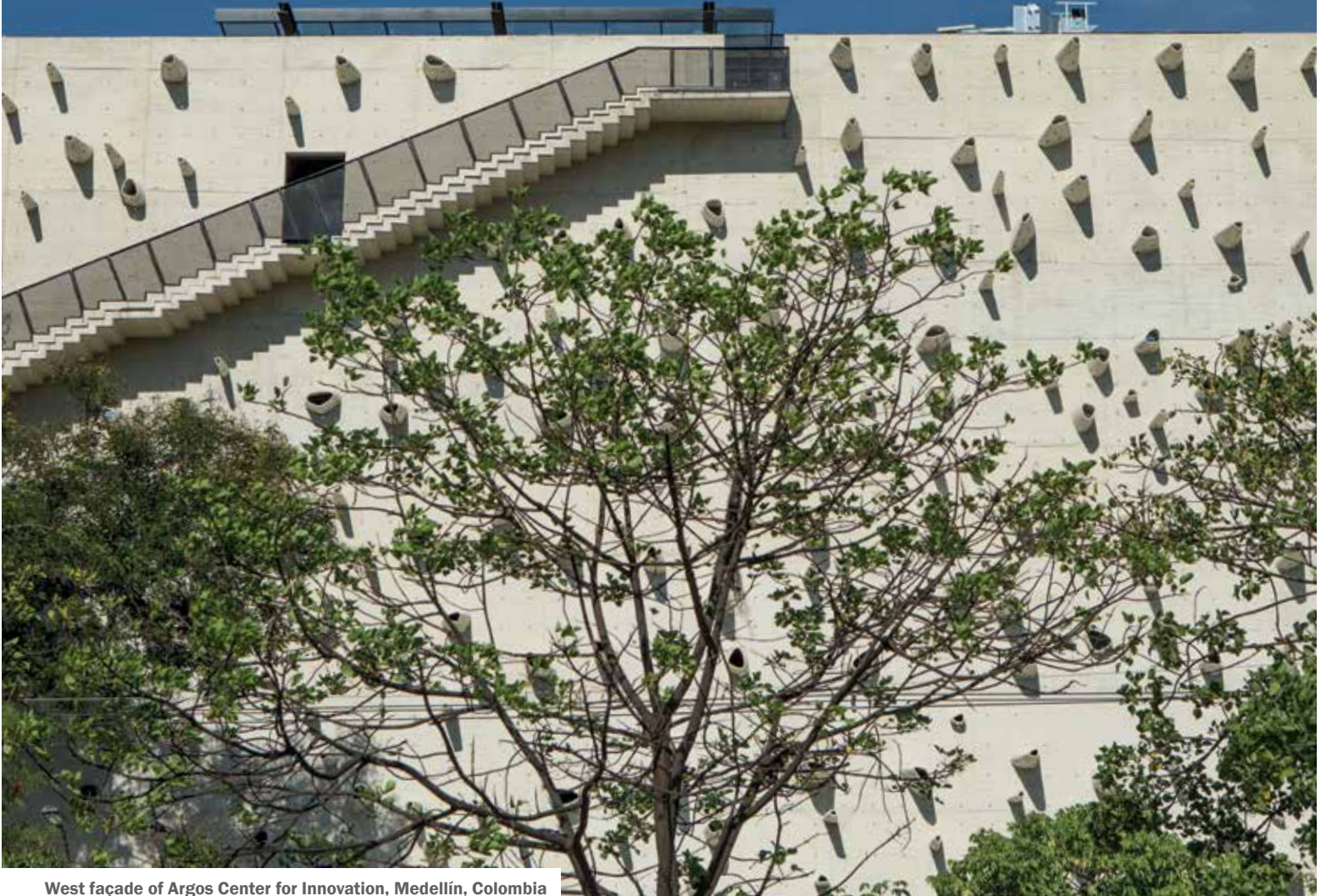
West façade of Argos Center for Innovation, Medellín, Colombia
