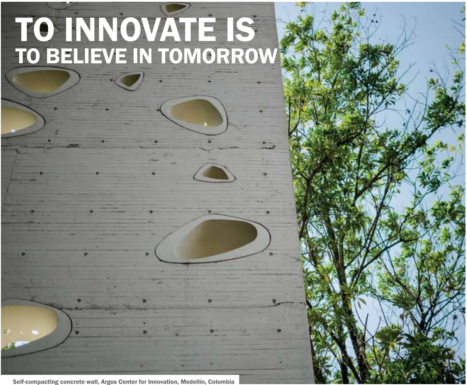
Self-compacting concrete wall, Argos Center for Innovation, Medellín, Colombia
