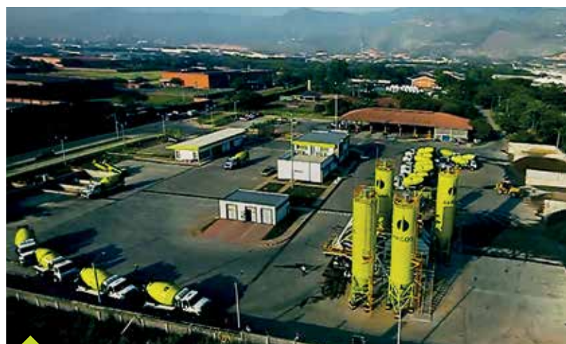
Arroyohondo Concrete Plant, Colombia Region
