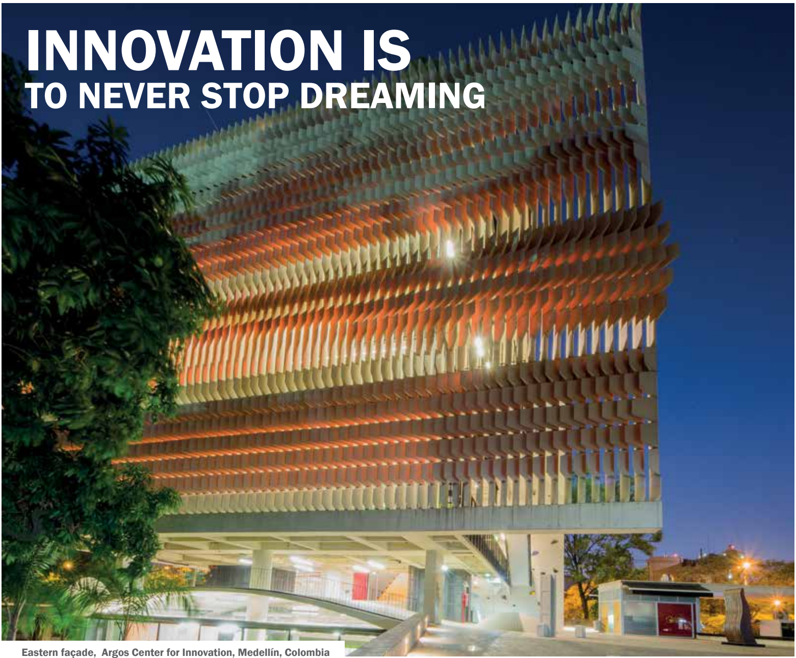
Eastern façade, Argos Center for Innovation, Medellín, Colombia
