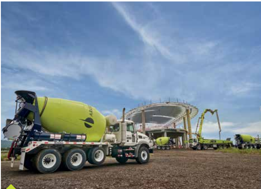
Tocumen International Airport, Panama
